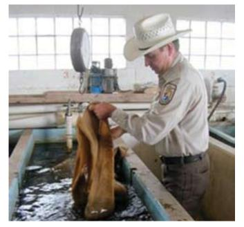
A U.S. Fish and Wildlife Service employee rinses a mesh "sock" that filters reservoir water entering the Inks Dam National Fish Hatchery, Texas. The sock keeps debris, fish eggs and fry from contaminating the hatchery's water supply and is an example of a "critical control point" designed to control aquatic invasive species introductions. Photo and description courtesy of the U.S. Fish and Wildlife Service, Inks Dam National Fish Hatchery and Minnesota Sea Grant.
