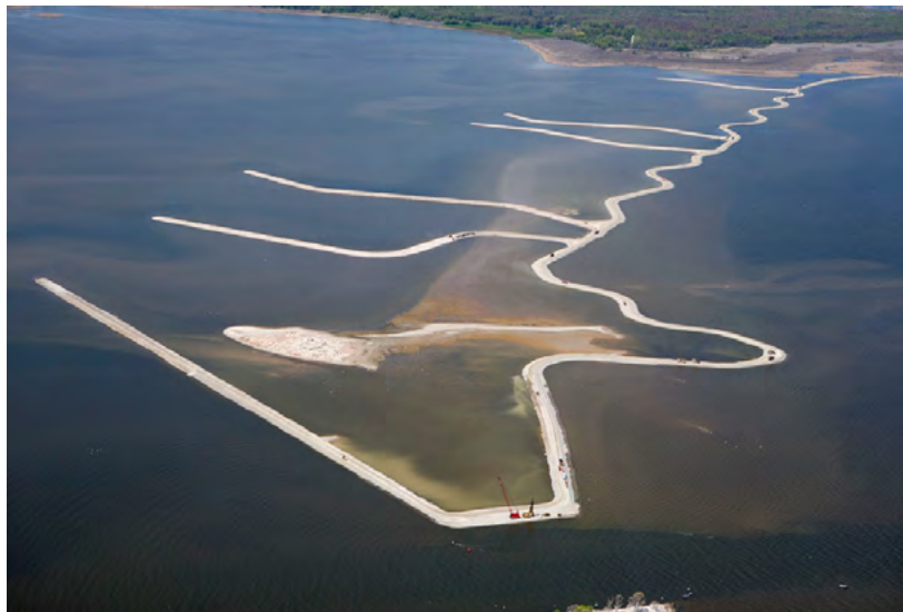
Figure 91: Cat Island spine construction, May 2013.
