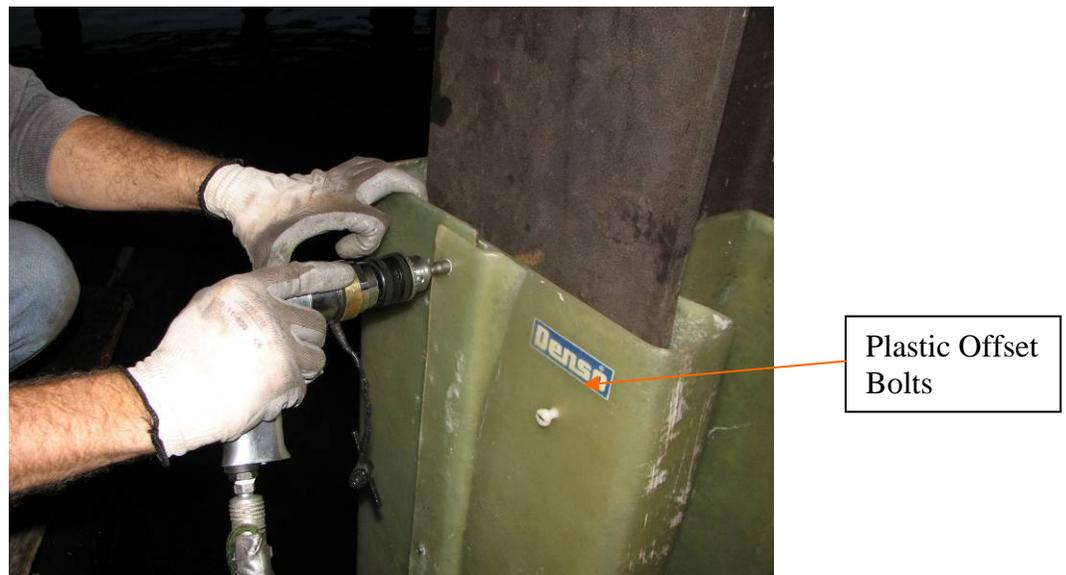
**Picture 7: 2-Pieces of Series 500 H-Jacket Being Fastened Together**
