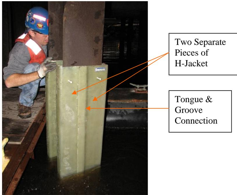
**Picture 6: Installing 2-Pieces of H-Jacket Around H-Pile**
