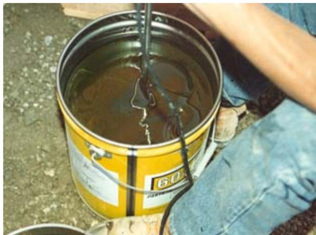
**Picture 9: Mixing SeaShield 550 Epoxy Grout**
