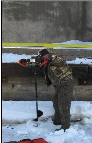
Individual holes were drills for each pipe and anode (ice was ~4 feet deep along pier).
