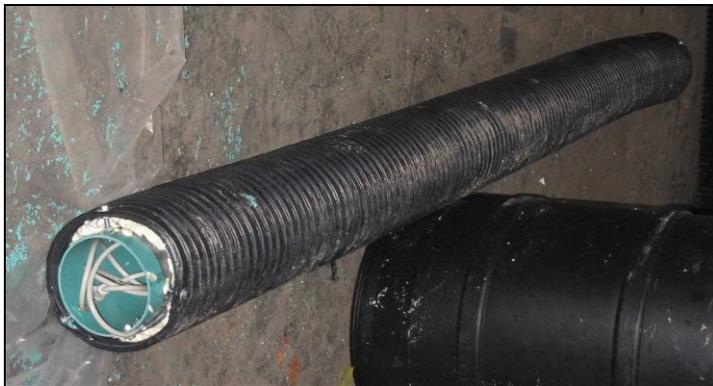
The 6" diameter pipe was then installed in and attached to an 8" corrugated PVC pipe (typically used for culvert installations). The top void between the two was sealed with expanding foam insulation to prevent heat loss from between the two pipes.
