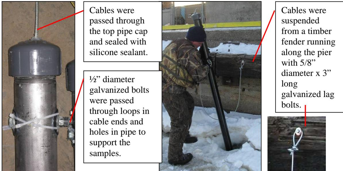
**Pictures 18 & 19: Pipe Sample Cable Support Installation**
