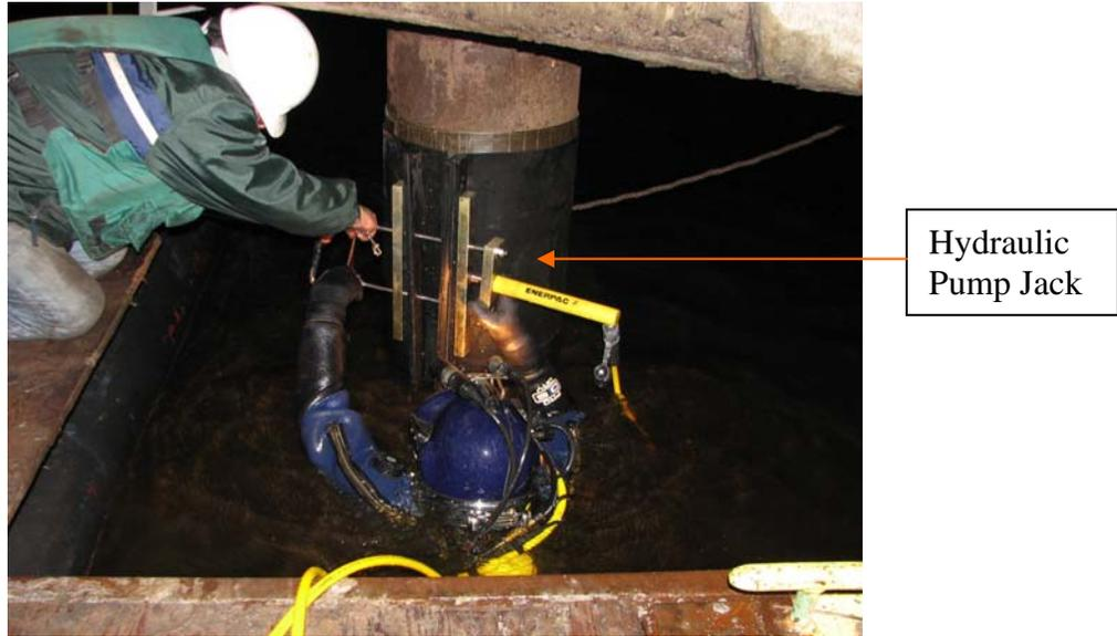
**Picture 3: Diver Installing Jacket with Use of Hydraulic Pump**
