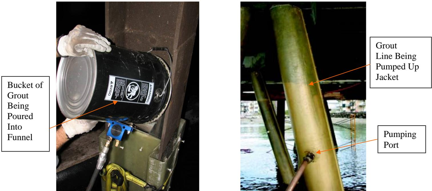
**Pictures 10 & 11: Placing SeaShield 550 Epoxy Grout**
