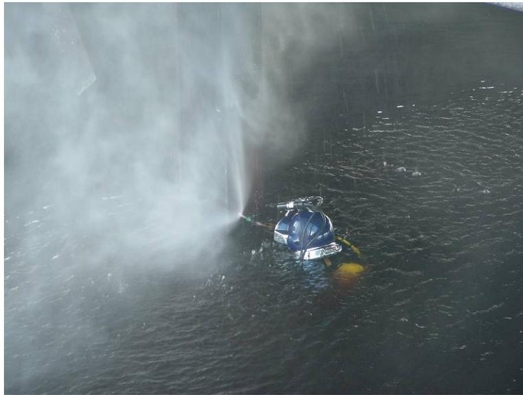
**Picture 1: Diver Performing Blast Cleaning**
