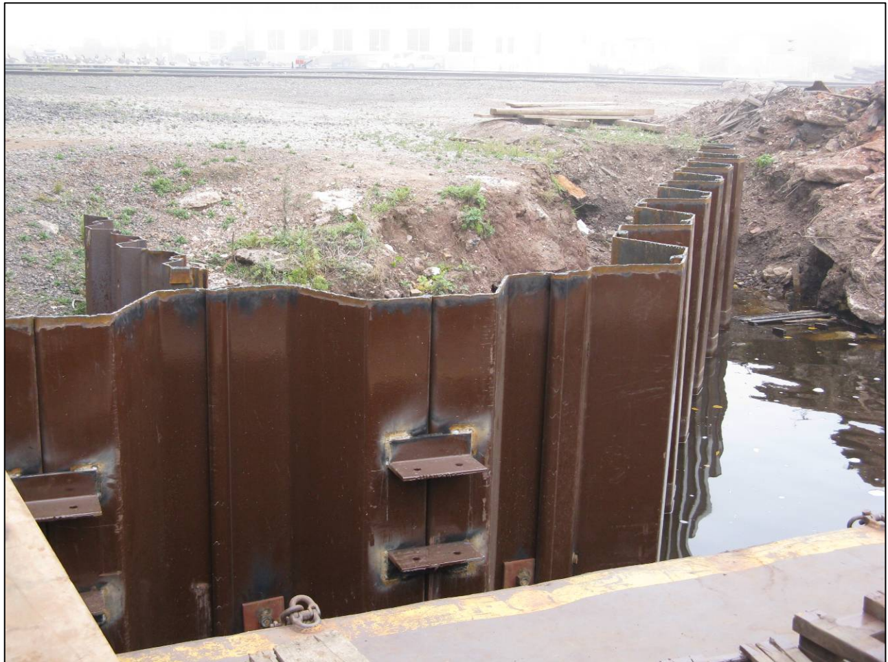
Picture 8: Newly installed sheet pile at Cenex Harvest States
