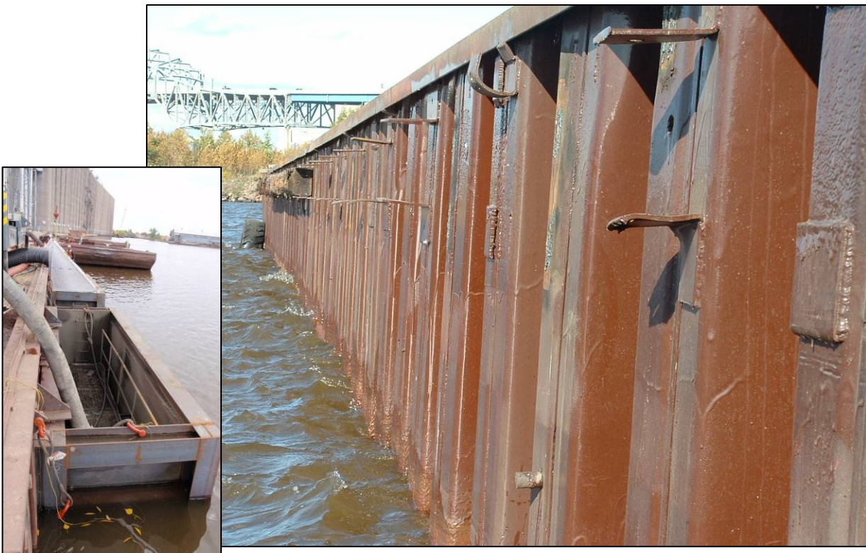
Pictures 6 & 7: Existing sheet pile at CHS was coated using a cofferdam
