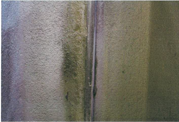
Picture 3: Angle iron used to seal an interlock.
