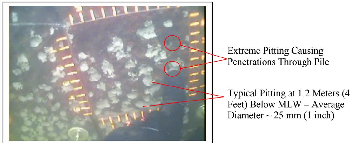
**Figure 1. Typical Sheet Pile Pitting and Penetrations**
