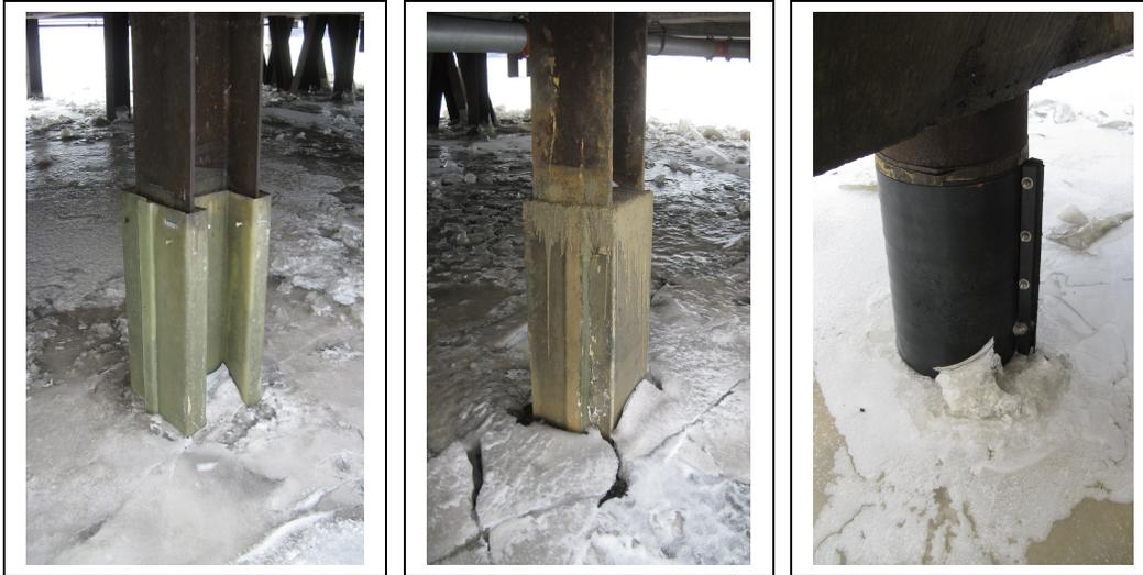
**Figure 8. H-Shaped, Rectangular, and Pipe Pile Protective Systems**
